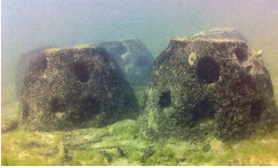
Rip rap or oyster reefs located just offshore of a marsh help to reduce the energy of waves hitting the coastline. Hollow concrete reef balls provide a manmade structure with functions similar to rip rap but designed to act as habitat for local fish and invertebrates. Under the right conditions, reef balls may encourage the establishment of oysters leading to an oyster reef. Photo credit: Reef Balls at Dutch Springs by Neil DeMaster, (CC BY-ND 2.0). https://www.flickr.com/photos/84169650@N07/10544449634 .
