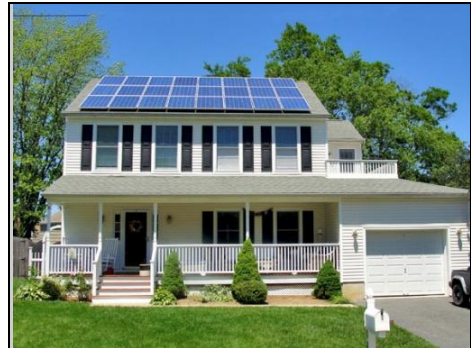
Residential Solar Panels
