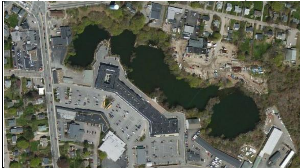
Example of Potential for "Non-Point Source" Contamination from Parking Lot Runoff
