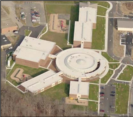
Community Facilities and Services
