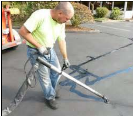
Sealing Roadway Cracks
