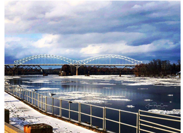
View looking north from Harbor Park
