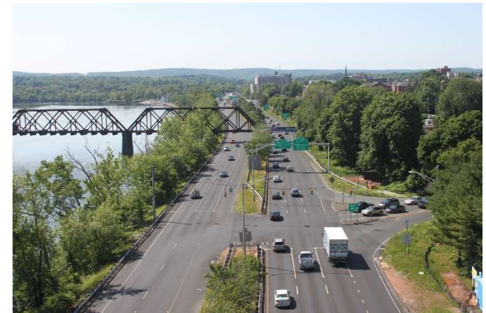
View looking south along Route 9
