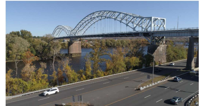
Arrigoni Bridge crossing the Connecticut River
