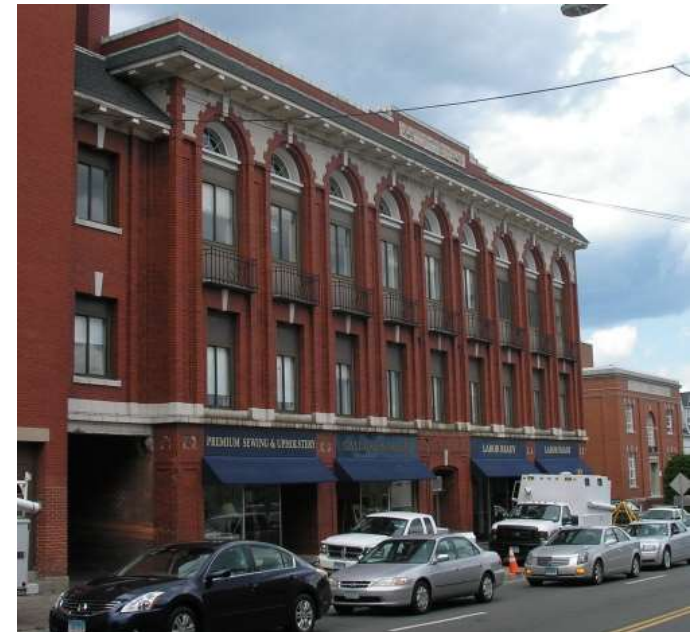
1890 building on Washington Street
