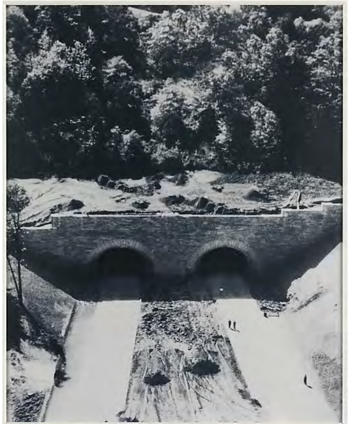
West Rock Tunnel, 1954 Photo: Robert Gober
