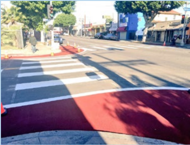
Figure 25: Example of a painted curb extension
