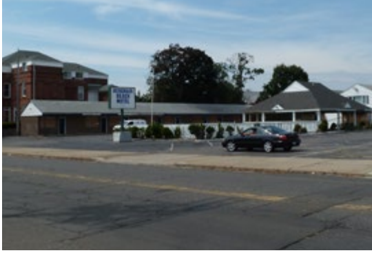
The vacant Debonair motel on Beach Street
