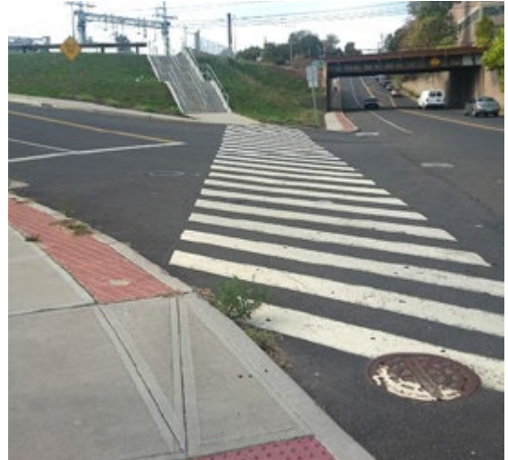
P-T4a. The intersection of Railroad Avenue and Saw Mill Road.
