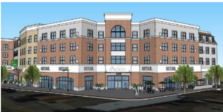
The Atwood, being constructed along Route 1 in Allingtown, represents a private redevelopment project stimulated by the growth of UNH. It will contain a total of 67 apartments (a mix of studios, 1 br, and 2br units) and 15,000 sf of ground floor retail space. This form, layout, and design of development is new for West Haven.
