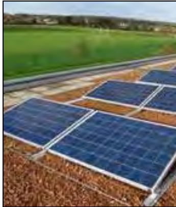
Rooftop Solar Installation
