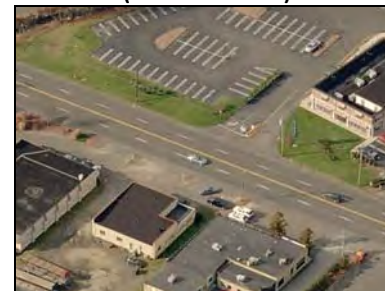
Older 4-lane Section (No Center Lane)
