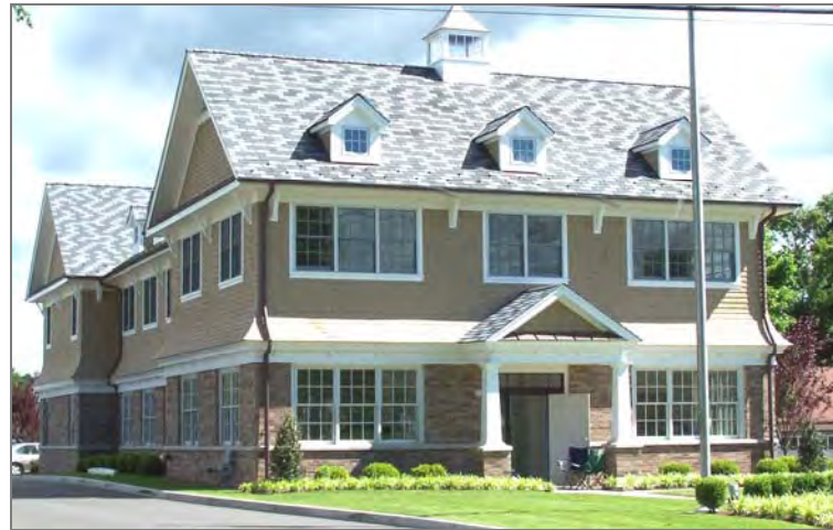
Many residents identified a new office building near Town Hall as the scale of building and type of architecture to encourage in this area.
