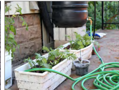
Rain barrels that store storm water for re-use.
