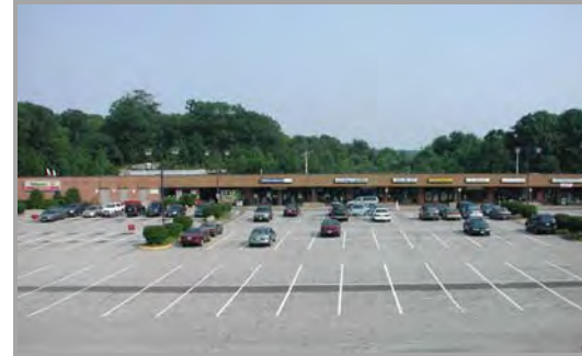
Strip style commercial site
