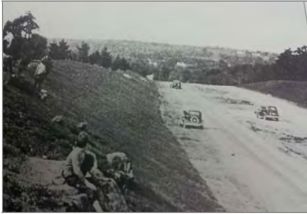
Construction of Merritt Parkway in Trumbull. 1935. Trumbull Historical Society.
