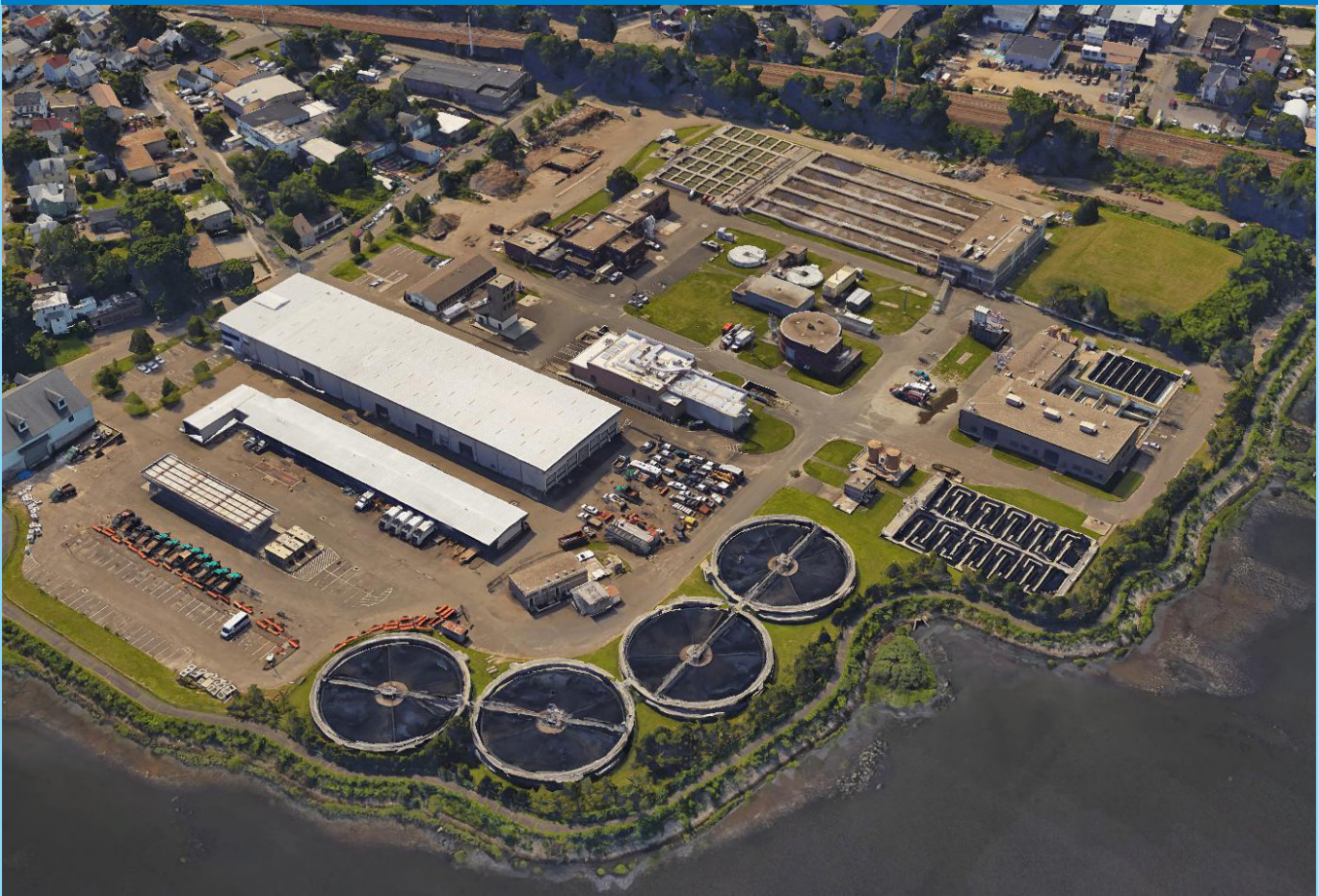
The Wastewater Treatment Plant at Liberty Point
