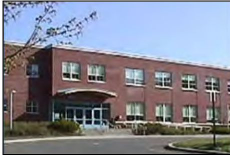
Royle Elementary School
