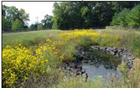
Water Quality Basin
