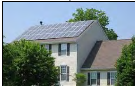
Residential Rooftop Solar Installation
