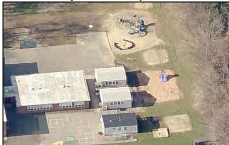
Portable Classrooms At Royle Elementary School
