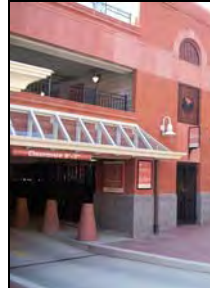
Unshielded Parking Structure
