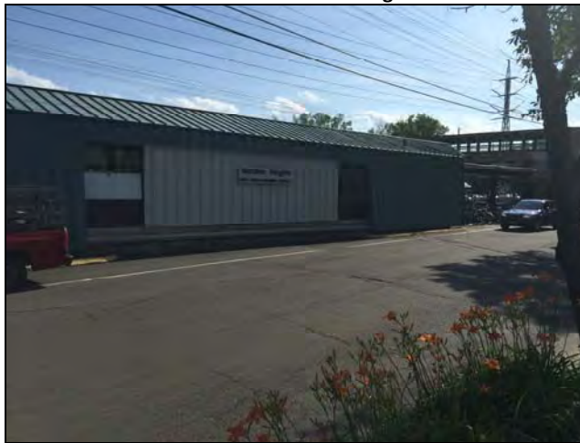
Existing Noroton Heights Train Station Building
