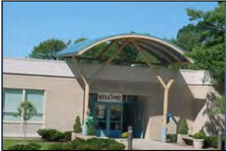
Ox Ridge Elementary School
