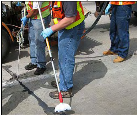
Crack Sealing
