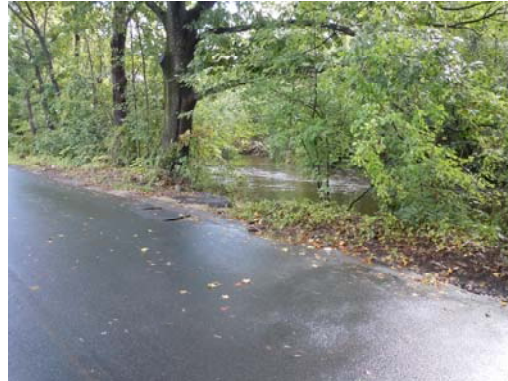
Area where Bladens River can flood roadways; note high flow of 9/8/12
