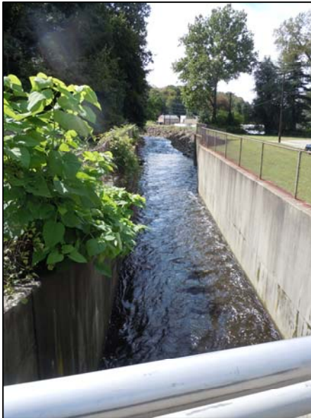
Section of flood control system in Ansonia
