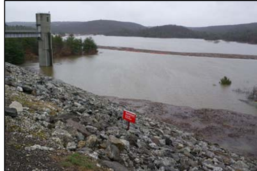
Thomaston Dam on Naugatuck River
