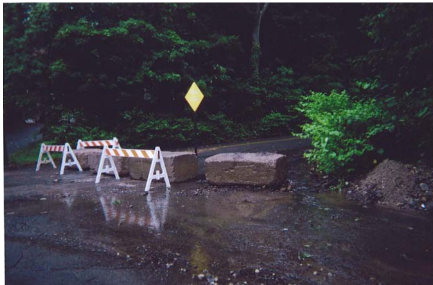
17. Northwest end of East Mountain Road (note flowing water)
