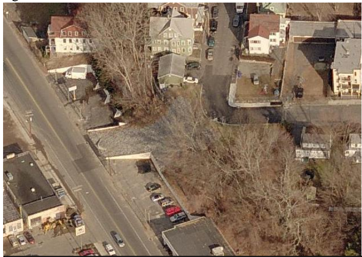
Site of slide between Southview Street & South Main Street
