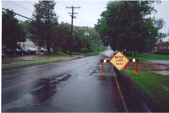
1. Warning sign on Sandbank Road in Cheshire
