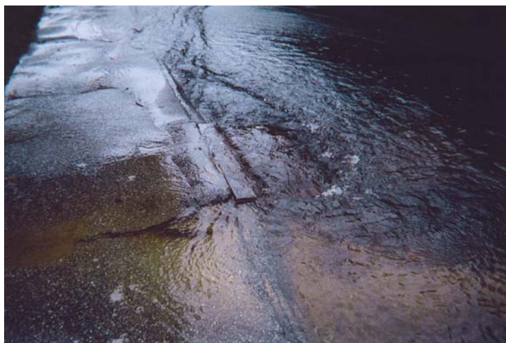
12. Water discharging from stormwater catch basin on Jersey Street
