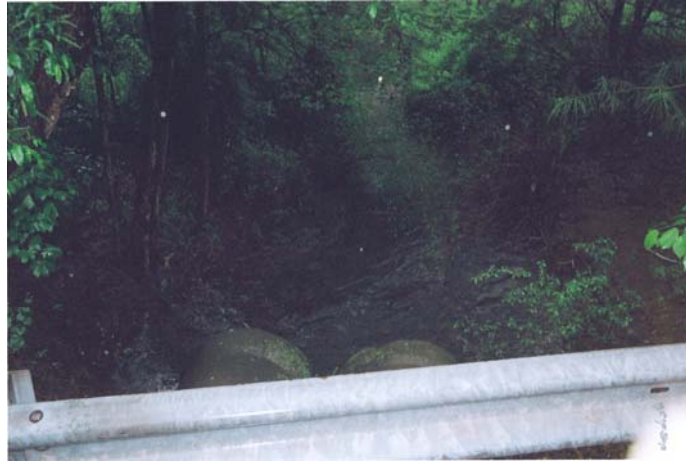
Honeypot Brook at East Gate Drive (note culverts)
