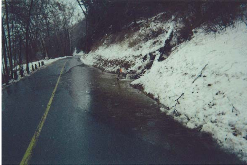
1. Nuisance flooding along River Road
