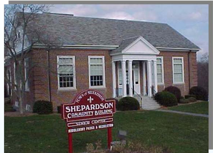
Shepardson Community Center is equipped with a generator
