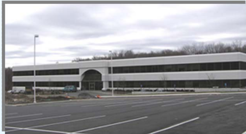
A mixed-use development located along Route 63 near Park Road. This development includes a large daycare center.
