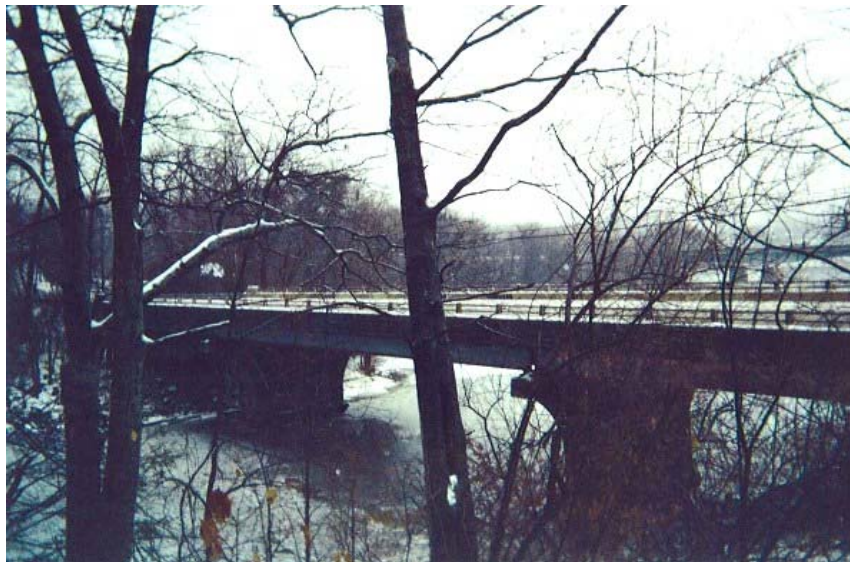
8. River Road Bridge over the Pomperaug River
