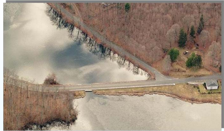
Long Meadow Road Bridge
