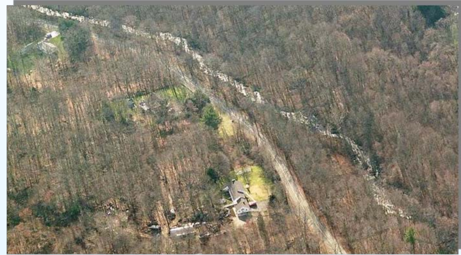
Regan Road runs parallel to Hop Brook south of Route 64
