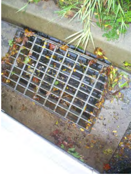
Photo 20: Storm drain adjacent to upstream culvert
