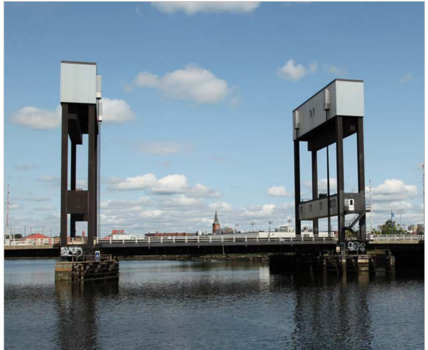
Route 130 over the Pequonnock River in Bridgeport. Source: M. Goetz
