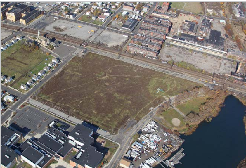
Site of the future Barnum Station Source: Barnum Station Feasibility Study, VHB
