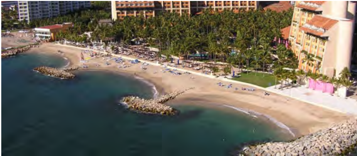
Figure 6 - Example of Offshore T-groins With Sand Deposit the Landward Side of the Beach
